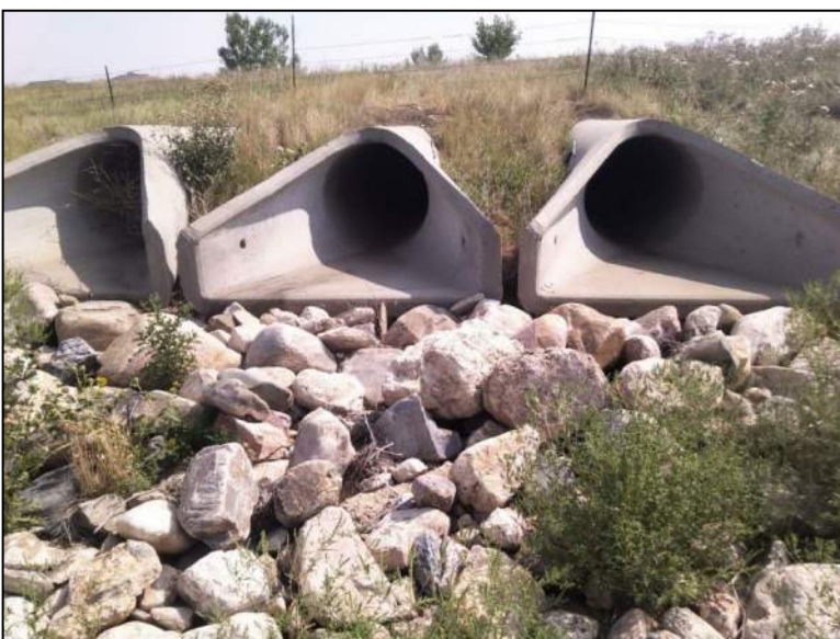
Photo 18: Culverts with Rip-Rap
